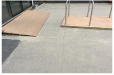
An additional layer of Wecryl 230 and Quartz Sand was added to provide extra protection and a key for the new paving slabs to be embedded.
