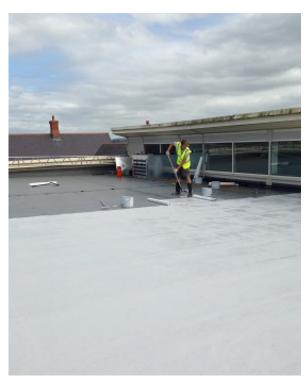
Direct wet on wet application method allowed a fast an efficient waterproofing system to be installed, with minimal disruption to the daily operation of the supermarket
