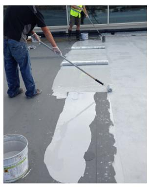
Waterproofing with Wethan 275 and reinforment in progress
