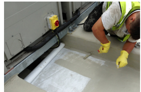
Further waterproofing of the details using Wecryl 230 thix.
