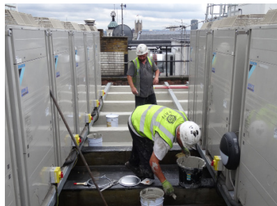
Plant Room Roof Area. Intricate details were easily waterproofed using Wecryl 230 Roof Waterproofing System
