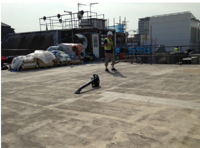
Existing Asphalt Roof Covering, correctly prepared and ideal to utilise as an existing substrate for Westwood Liquid Technologies Roof Waterproofing Systems
