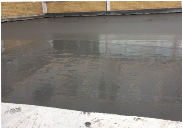
The Wecryl 230 reinforced waterproofing being applied
