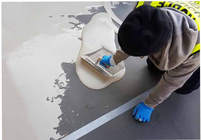
The Wecryl 233 wearing layer applied using a trowel with the quartz sand broadcast to follow
