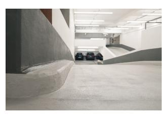
The Weproof High-Build System proved an excellent choice as a protective, heavy-duty wear layer. A special characteristic of this system is that it possesses the necessary SBauVO approval as regards its reaction to fire.
