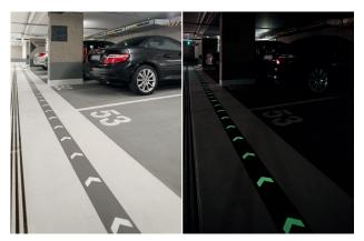
PMMA-based products were also used for marking the escape routes, although in this case with afterglow additions. This means that customers can safely find their way out in an emergency, even in the dark.
