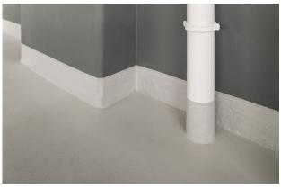
The fleece-reinforced, liquid waterproofing system, classified as flame-resistant, incorporates all upstands and details up to a height of 15 cm, thereby providing reliable protection against moisture and chloride.
