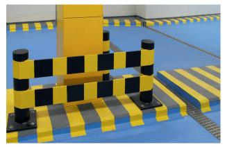
The drainage channel across both lanes is securely integrated in the fleece-reinforced waterproofing system.
