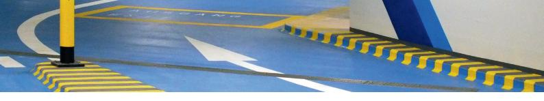
Car park design featuring PMMA liquid waterproofing system
