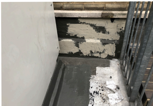
Weseal 810 Putty was used for uneven surfaces
