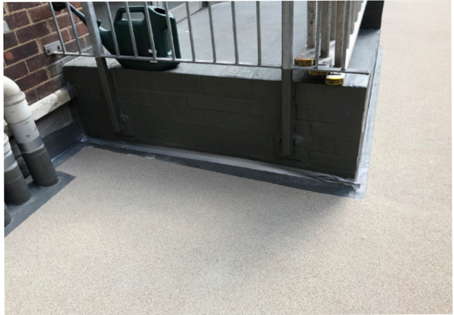
Wecryl 233 wearing layer with a quartz sand broadcast was added to the hardstanding area.
