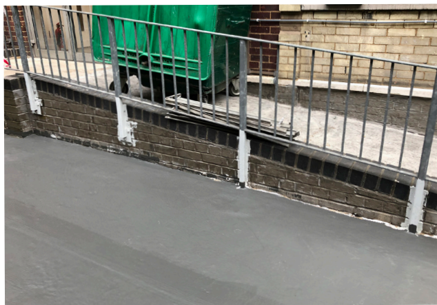
Weseal 815 Fibre Putty was used for awkward and fiddly detailing
