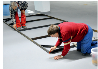
The bays are measured out and masking tape is applied exactly in line with the layout
