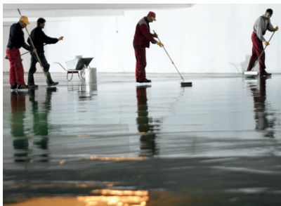
Weproof Fix RR 359 in green, a waterproofing product for main areas, is applied using notched trowels and spiked rollers
