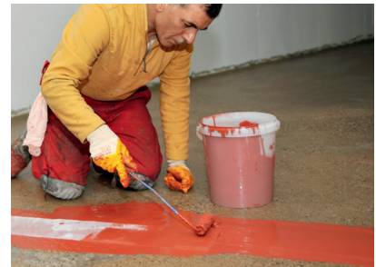
This involves applying an initial layer of PMMA resin, embedding the strips of fleece and removing any air bubbles, then saturating the fleece with the same resin
