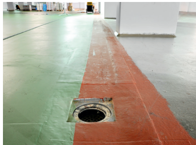
Details on gullies and floor drains are waterproofed wet in wet with Weproof Flex RR 354 and strips of WestWood Fleece
