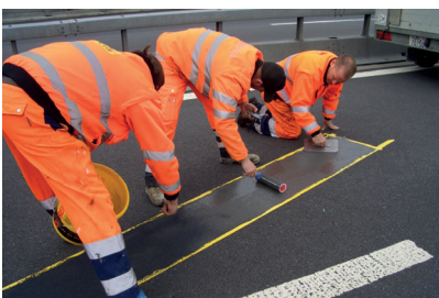
5. Wecryl 420 Rolled Surfacing is dressed with a hard topping, grain size 0.6 to 0.9 mm, and the motorway pavement is fully reinstated
