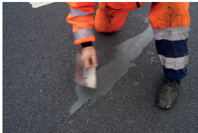
2. The damaged sections are cleaned and then filled with Wecryl 242 Mortar or Wecryl 420 Rolled Surfacing
