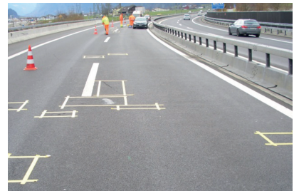
3. The patches are marked and then concrete masking tape is applied to the edges
