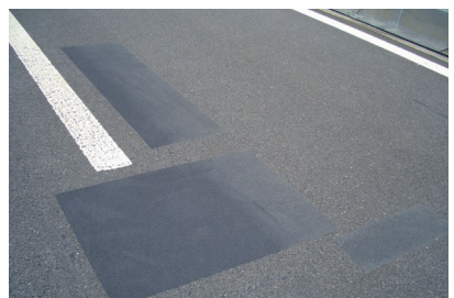
6. The patches can be walked on after just 45 minutes and the road is soon ready to be reopened to traffic
