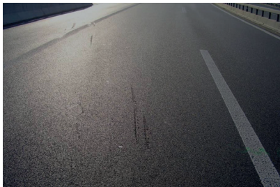
1. Superficial damage to the MR8 pavement. The damage is 5 to 30 mm deep
