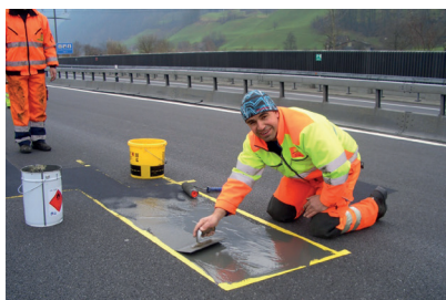
4. Wecryl 420 Rolled Surfacing is applied with a trowel and roller, incl. surface dressing
