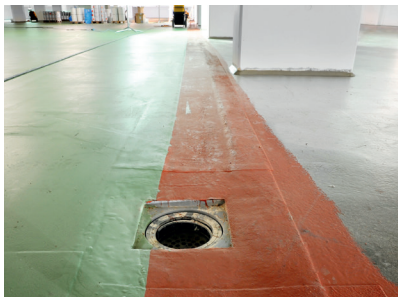
Details on gullies and floor drains are waterproofed wet in wet with Weproof 264 and strips of WestWood Fleece
