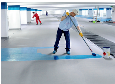
The parking bays are sealed with low-maintenance Wecryl Finish 288 in shades of green and blue
