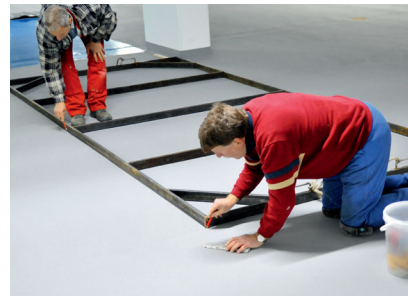
The bays are measured out and masking tape is applied exactly in line with the layout
