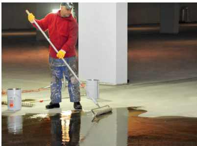
Wecryl Primer 276 is applied to the shot-blasted concrete surface
