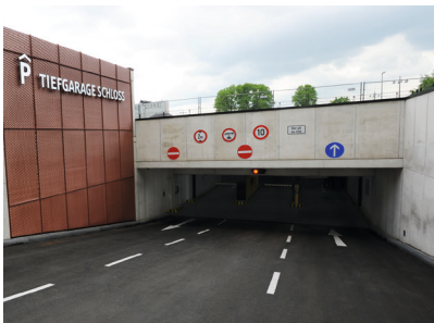
Schloss underground car park, Koblenz (CPS)
