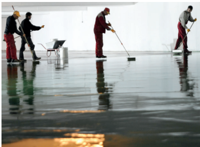
Weproof 269 in green, a waterproofing product for main areas, is applied using notched trowels and spiked rollers
