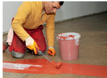
This involves applying an initial layer of PMMA resin, embedding the strips of fleece and removing any air bubbles, then saturating the fleece with the same resin
