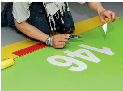
Stencils are used for applying the bay numbers...
