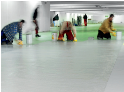
Stainless steel trowels are used to apply hard-wearing Wecryl textured surfacing
