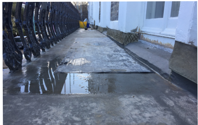
All areas were made watertight using Wecryl 230/230 Thix & Fleece
