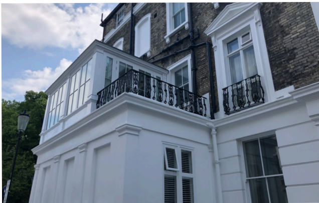
Balcony area that forms a roof above the dwelling below which also received a tile effect waterproof system.
