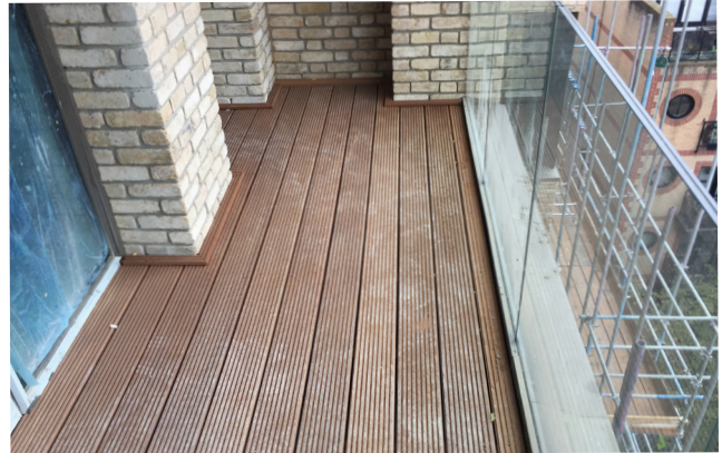
Decking installed on top of the waterproofing
