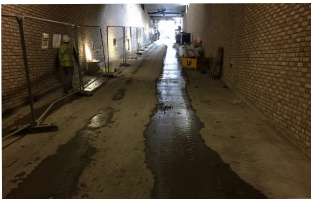
The access ramp required waterproofing prior to the hot rolled asphalt being installed
