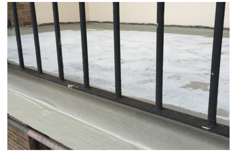
3. Waterproofing - Wecryl 230thix
