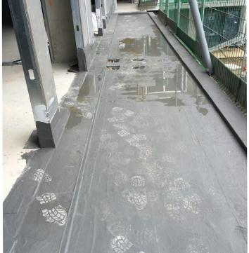
**Background:** Parkside Place is a substantial new build development with numerous balconies that required waterproofing in an efficient manner whilst other trades were present on site.
