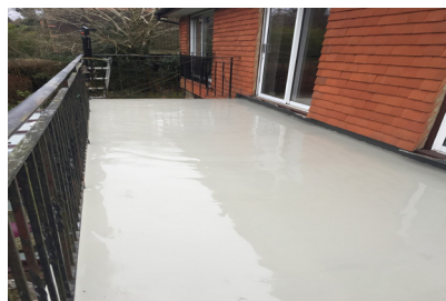
2. Continued with Wecryl 230 Waterproofing & Wecryl 233 Protective Layer
