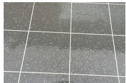
3. Finished refurbished balcony with a Wecryl 288 Tile Effect Layer using deco chips as additional slip resistance
