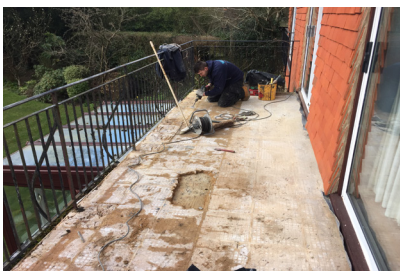
1. Balcony prior to any preparation work and cleaning ready for the priming and waterproofing to commence
