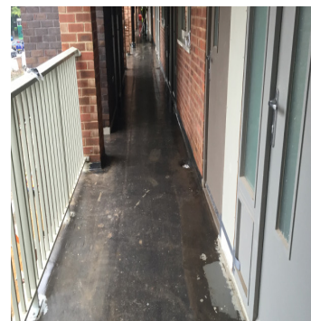
Walkway cracks and gaps sealed using Weseal 815 Rapid Curing Mortar
