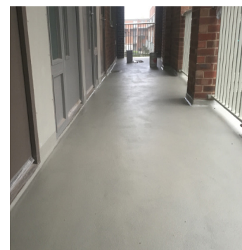
Walkway successfully coated & waterproofed with rapid curing Wecryl High Build System
