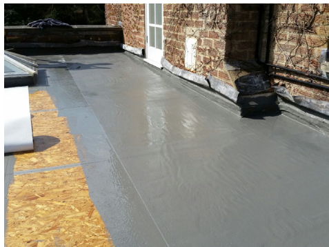
Wecryl 230 Waterproofing Layer being installed with reinforced Fleece.
