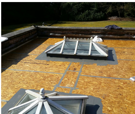
Board joints and upstand details completed with Wecryl 230thix Waterproofing Layer + reinforced Fleece. Ready to start on field area.
