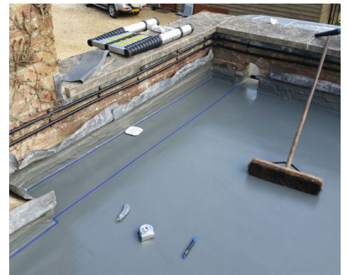
Grout lines being taped out on Waterproofing and Hard Wearing Layer. Ready for a tile effect Finish with black/white Deco Chips.
