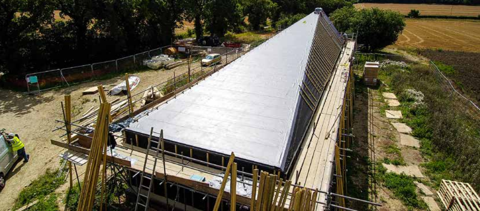
DANOPOL® WATERPROOFING COMPLETED
