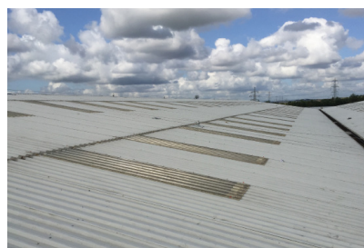
1. Roof Lights coated with Wecryl 220 Translucent Sealer to inhibit UV and Infra - red degradation
