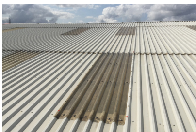
1. Roof Lights coated with Wecryl 220 Translucent Sealer to inhibit UV and Infra - red degradation
