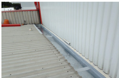
2. Canopy roof prior to coating
