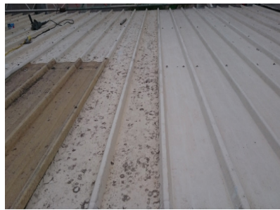
All the dirt and flaking paint needed removing and any shiny galvanized metal had to be abraded prior to coating. The left panels reflect the uncleaned area compared to the cleaned ones on the right
