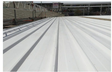
Wecryl 288 Finish in White was installed on the plastisol sheets to enhance and protect. Covered by our WestWood insurance backed Warranty
