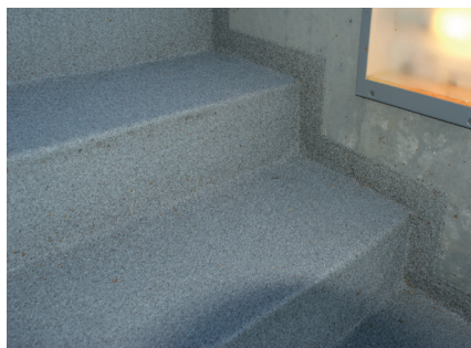
Weplus Coloured Quartz with Wecryl 220 transparent sealer
