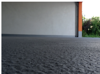
Wecryl 420 roller-applied coating
