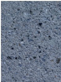
Surface after bush-hammering
