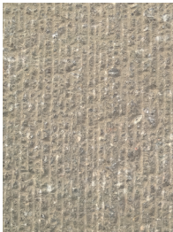
Surface after scarification
