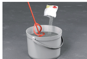
3. Add the catalyst (according to mixing table, temperature and application time) and mix for 2 minutes with a slow-speed stirrer. (Small amounts may also be mixed manually.)
